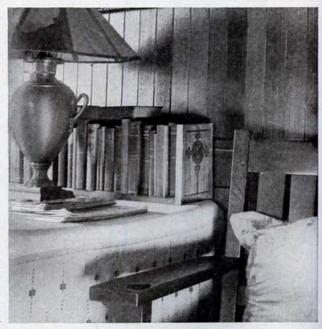
rack is left in the natural soft wood color, the whole being treated to two coats of orange shellac. It has held the working books of four children as they went through the grade schools and on to college. Its construction is so simple as to need no special directions as to details. The back-board is let into the end pieces by means of a half-lap joint, nailed, and the base is nailed to the ends.
